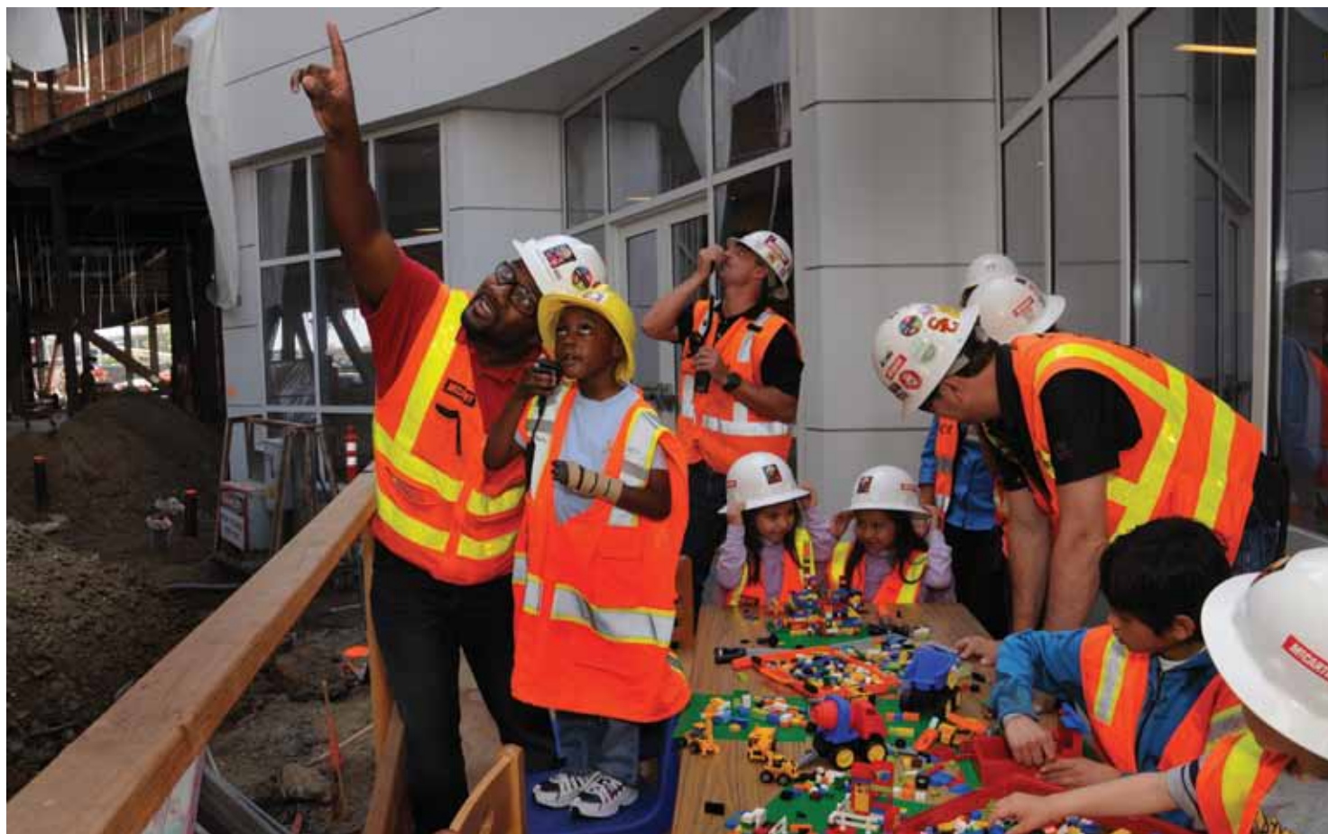
With construction of Torrance Memorial Medical Center's nearly 400,000-square-foot new Patient Tower happening in the background, Pediatric Burn Unit patients teamed up with workers from McCarthy Building Companies, Inc., to create their own rendition of the new hospital building using LEGOS®. Seen here is John Sanders guiding 5-year-old Robert Jones, who has been undergoing treatment for burn injuries at Torrance Memorial Medical Center, to make the command to complete the final seventh-floor cement pour in the new Patient Tower. Sisters, Litzzy and Karime Santos also participated in the mini building project, along with other Pediatric patients. McCarthy donated several sets of LEGOS® to the Pediatric Unit to help keep young patients entertained during their hospitalization. Photo by Deidre Davidson.
